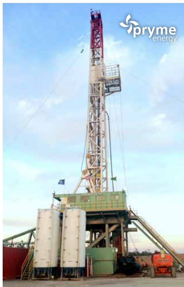
Drilling begins on the Rosewood plantation 21H well
